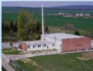
Radioactive Waste Management - in Püspökszilágy
