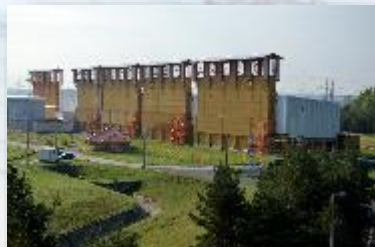
Spent fuel interim storage facility
